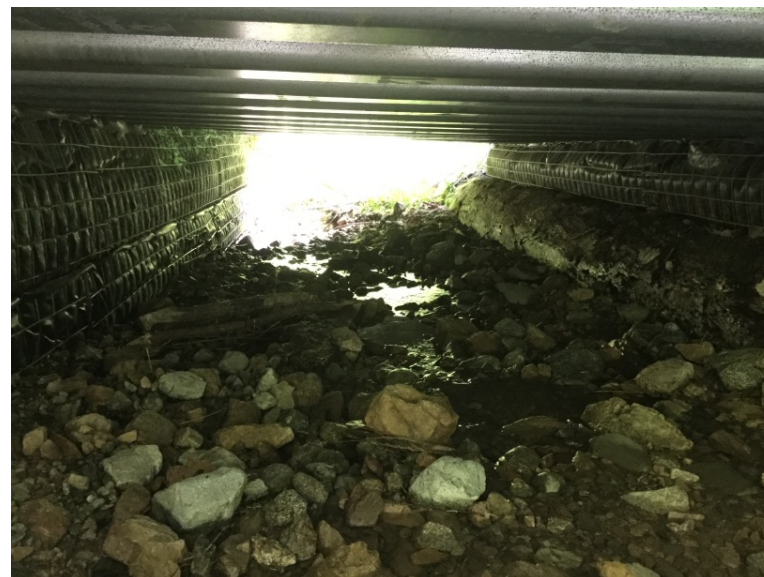
Looking through from inlet
