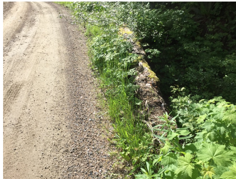
Upstream log curb outside wire mesh forms
