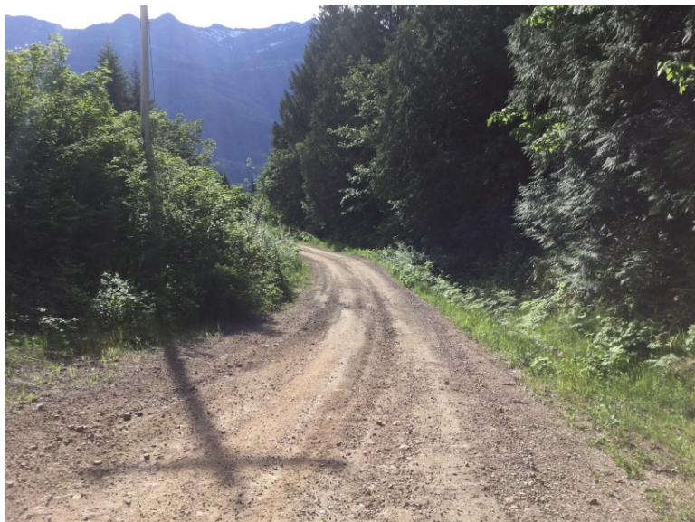
Approach from Left Bank when facing downstream
